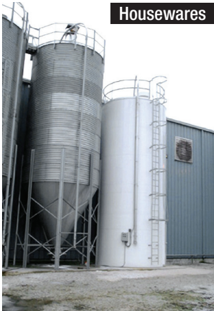
Bolted corrugated silos
