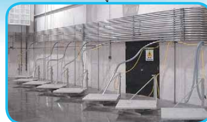
Tilt Tables and Piping
