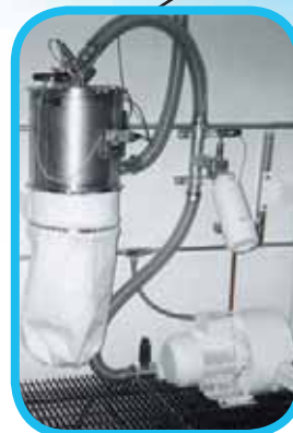
Vacuum Pumps and Central Filters
